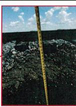
Shows depth of hole created by collapsed drainage culvert.
